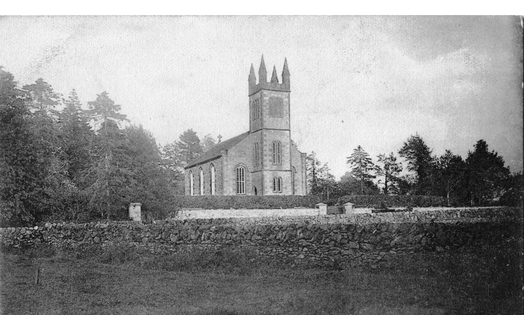
ANWOTH PARISH CHURCH, GATEHOUSE-OF-FLEET.
